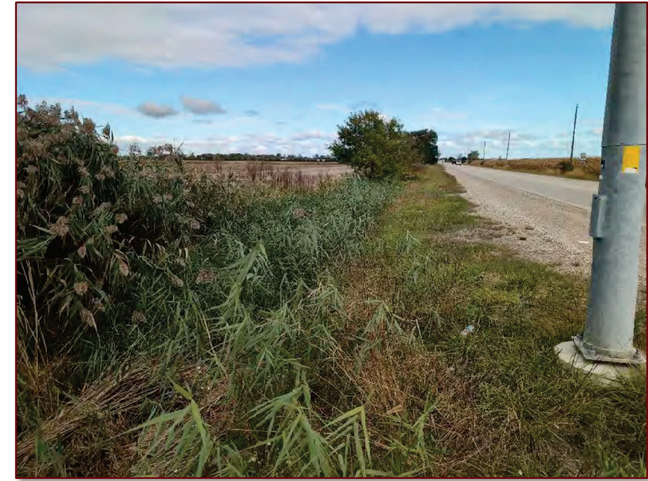
Image 22: 9 th Concession Road – Drain and Raised Road Bed
