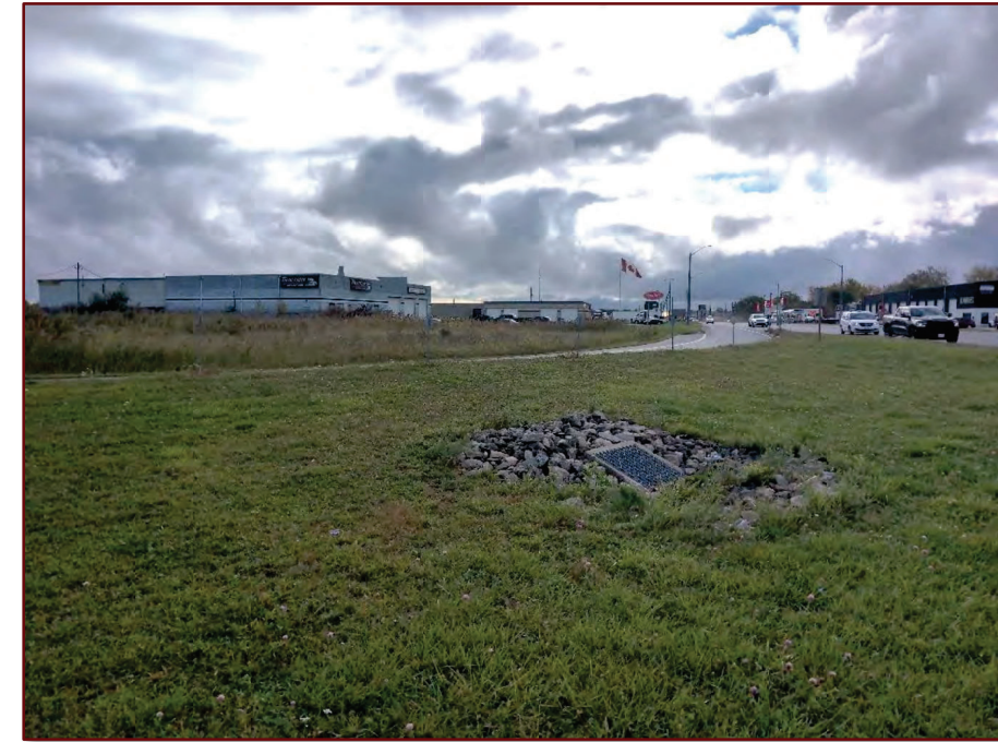
Image 2: County Road 46 – Above and Below Ground Utilities, Landscaped Areas
