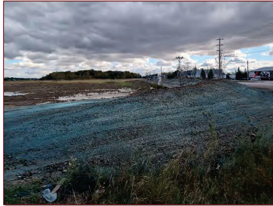
Image 12: County Road 46 – Ditch, Utilities and Paved Areas
