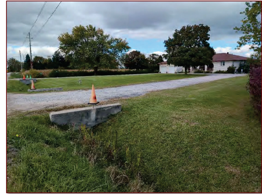
Image 34: County Road 46 – Gravel Laneway, Structure, and Utilities
