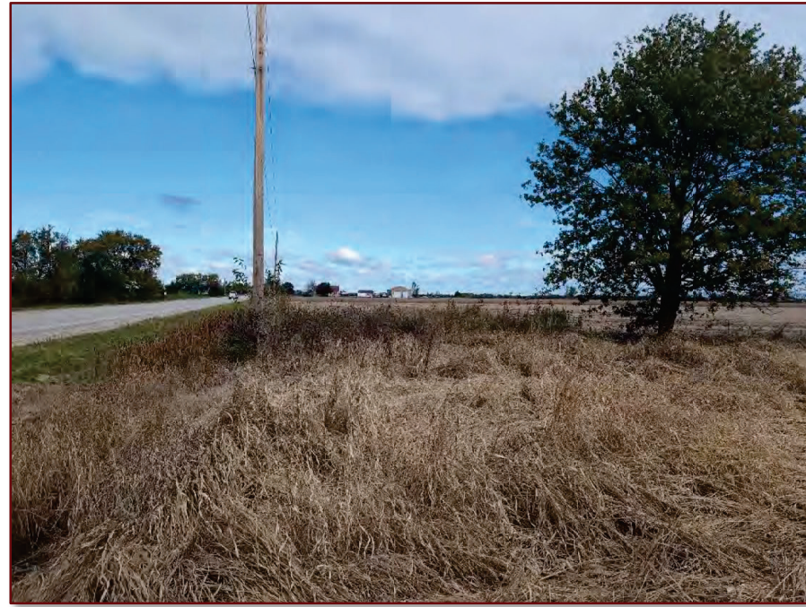
Image 24: 9 th Concession Road – Raised Roadbed for Highway 401 Overpass
