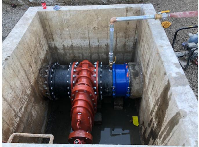
New 24" Horizontal Gate Valve in a concrete chamber at the intersection of California and College.
