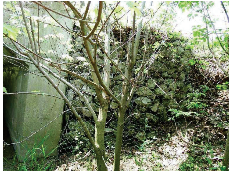
Figure 14 - Northwest Embankment/Slope Protection
