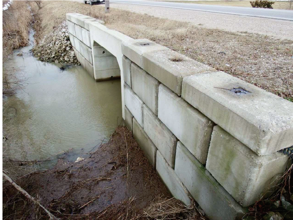
Figure 3 - South Headwall/Curb
