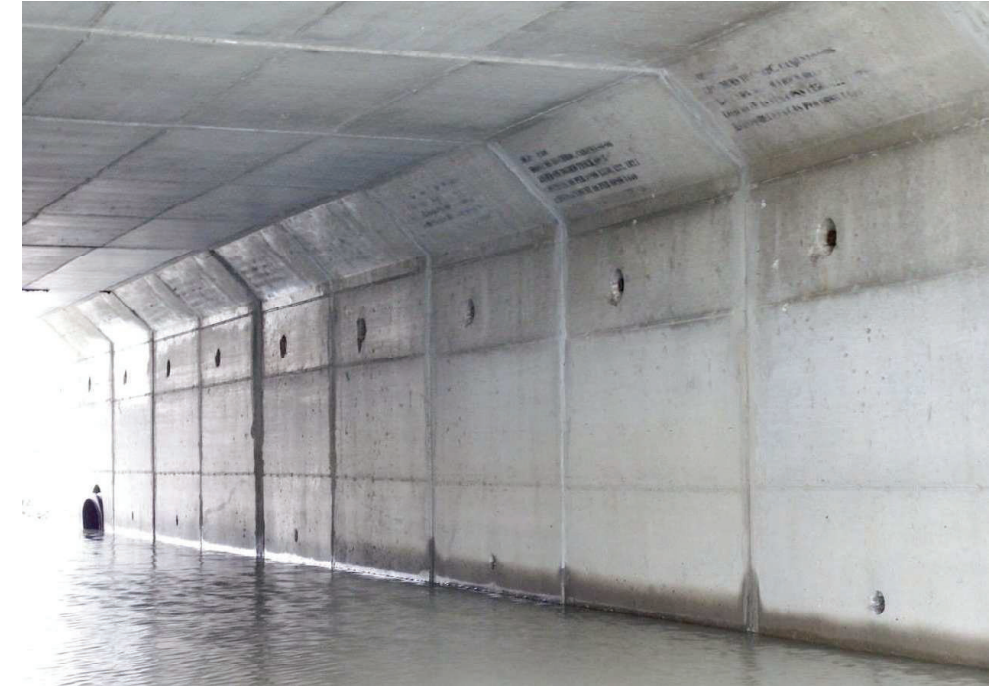
Figure 5 - Abutment Wall (Looking North)
