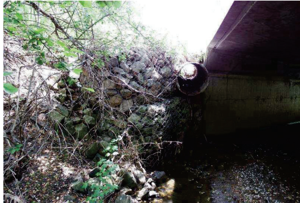
Figure 13 - Northeast Embankment/Slope Protection
