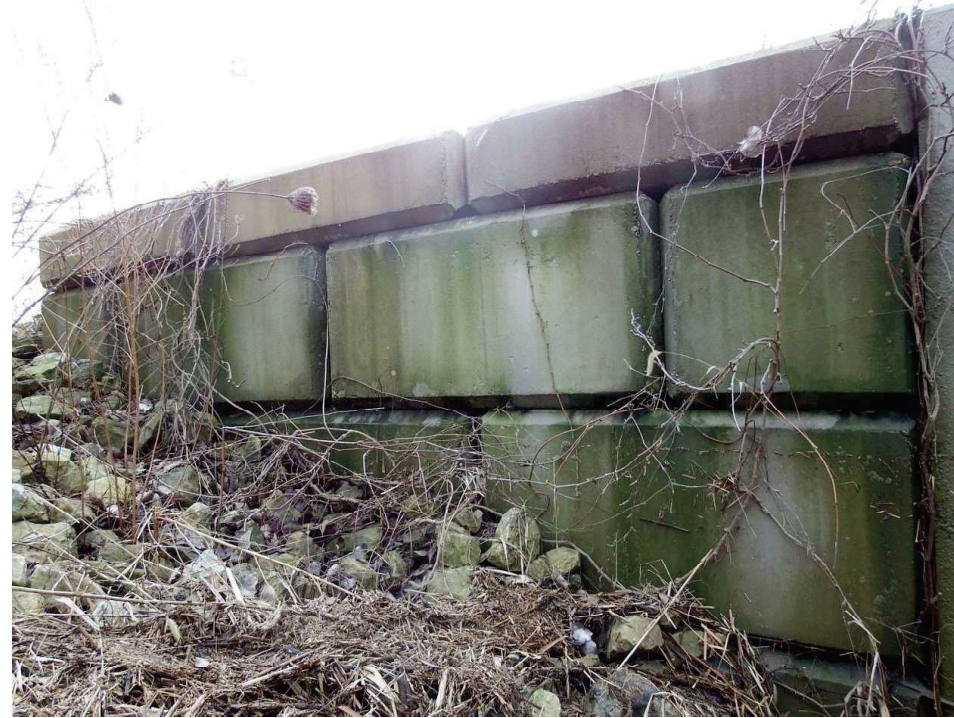
Figure 7 - NE corner of Headwall
