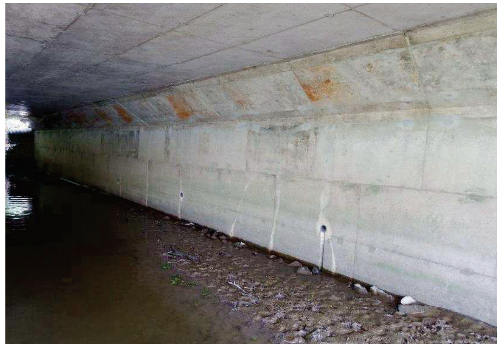
Figure 6 - East Abutment Wall
