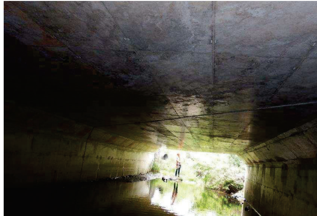
Figure 9 - Interior Soffit Looking South
