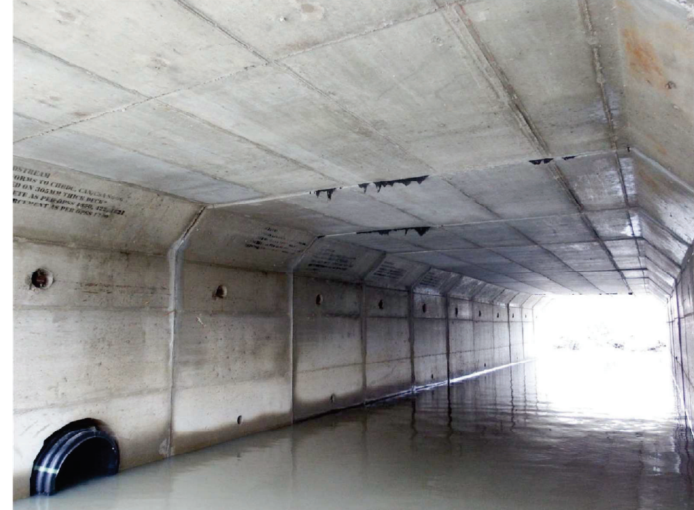
Figure 9 - Culvert Barrel (Looking South)
