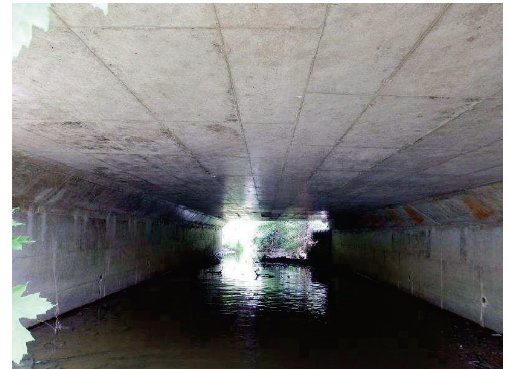
Figure 4 - Interior Soffit Looking North
