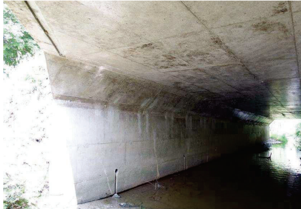
Figure 5 - West Abutment Wall
