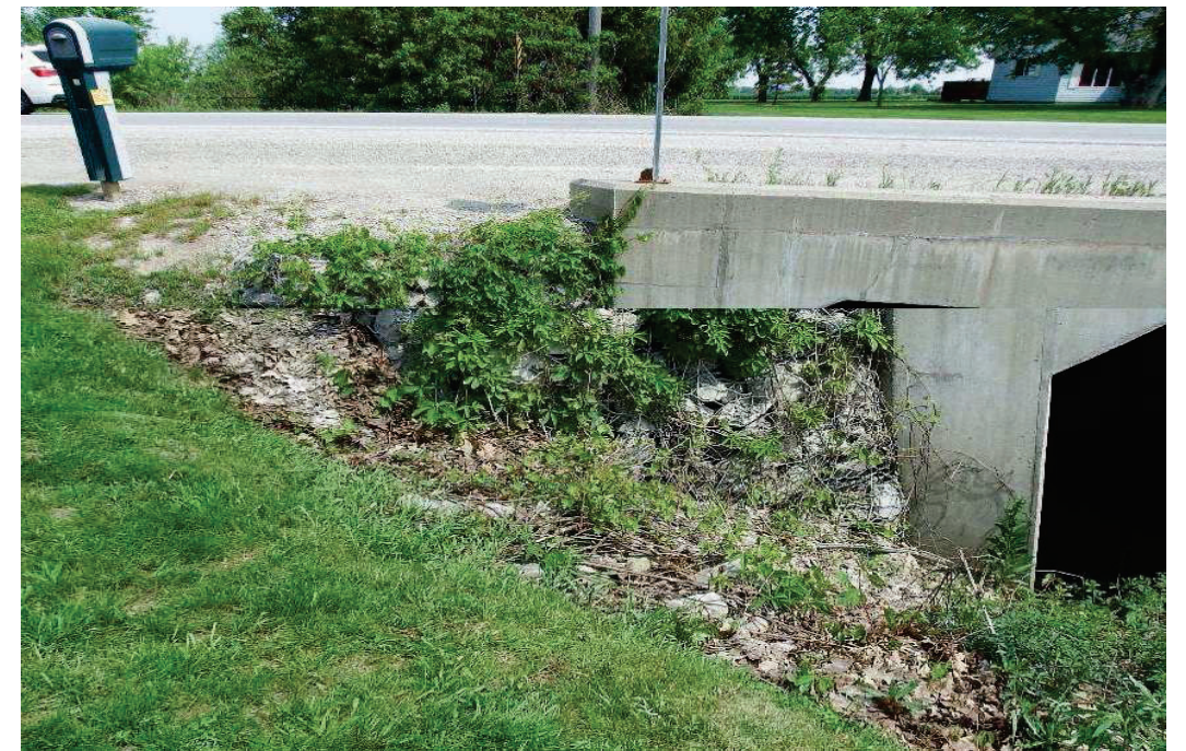
Figure 12 - Southwest Embankment/Slope Protection
