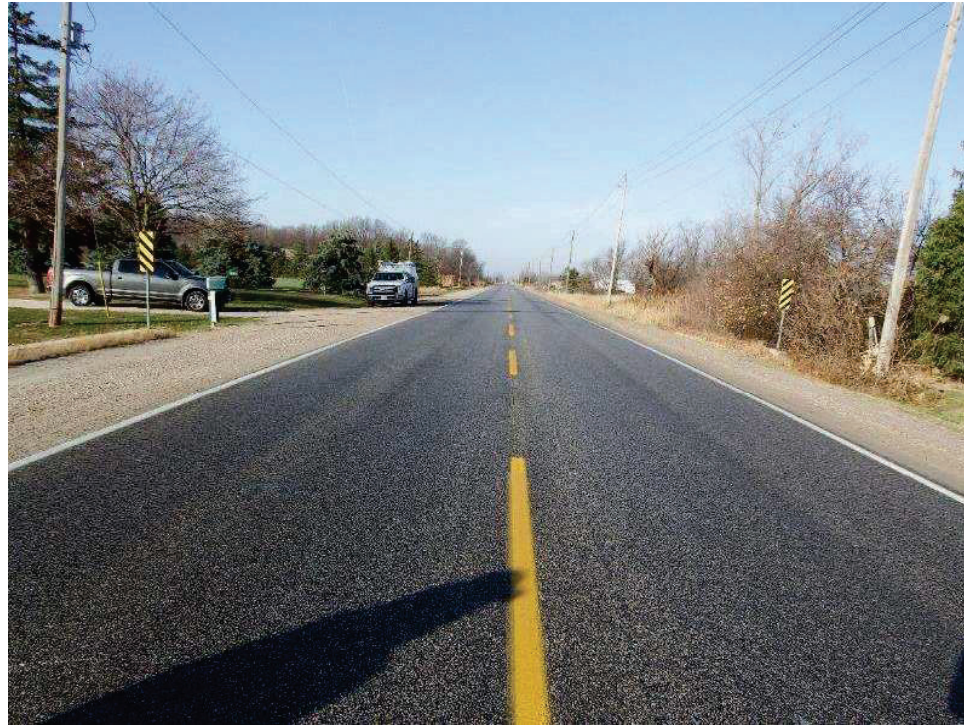
Figure 1 - Asphalt Wearing Surface Facing West
