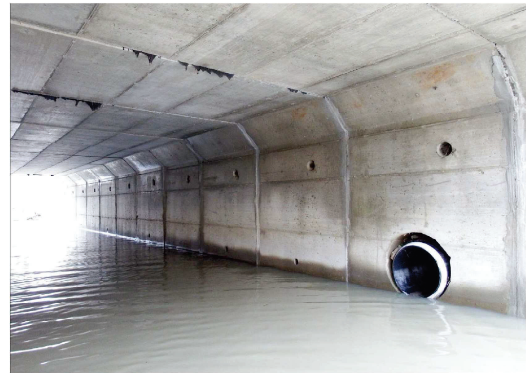
Figure 10 - Culvert Barrel (Looking South)
