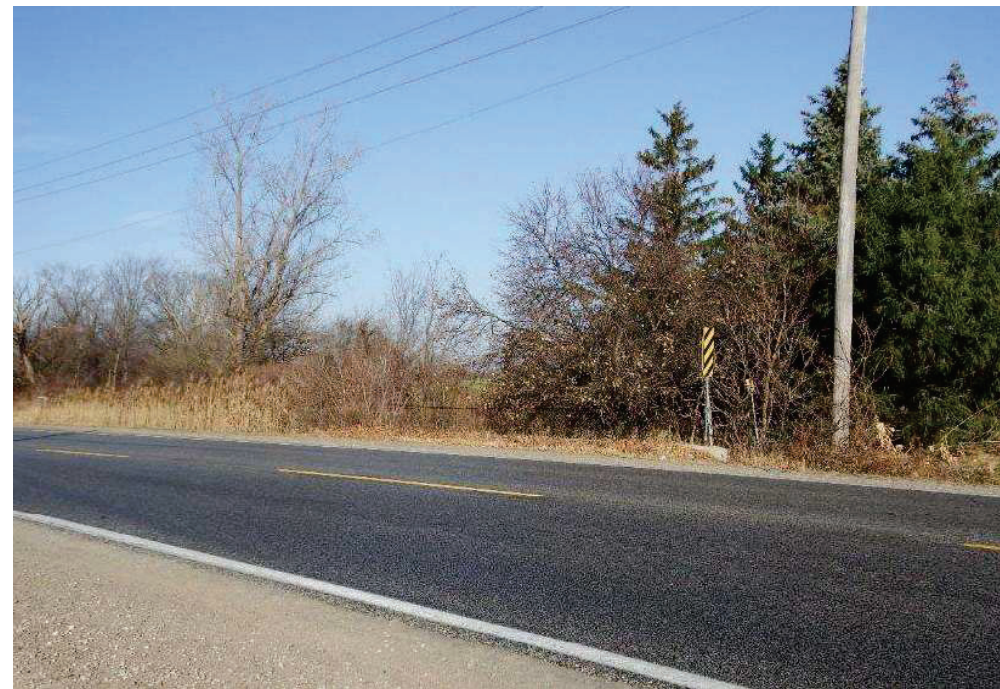
Figure 2 - Asphalt Wearing Surface Facing North
