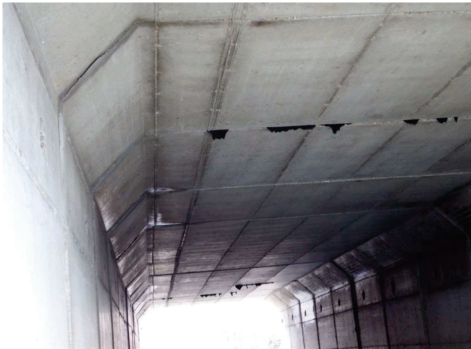
Figure 4 - Interior Soffit (Looking North)
