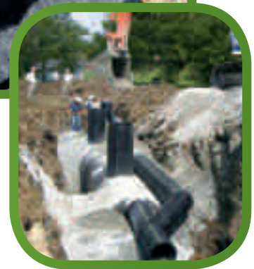
A bypass system (above right) is installed to prevent water flows greater than the first flush from re-suspending captured pollutant particles.
