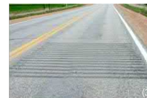
Rumble strip Vertical deflection; Small bumps in the roadway surface causing vibration in automobiles
