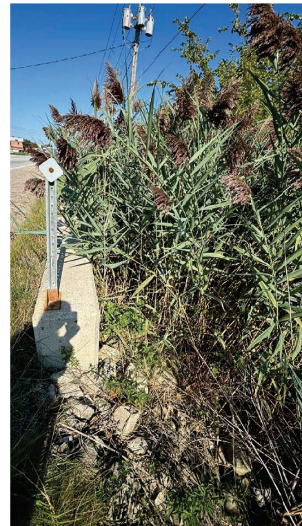
Photo 8: Facing west at Crossing 3, from the north side of County Road 46.
