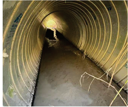
Photo 34: West barrel of concrete pipe culvert at Crossing 6 (facing south).
