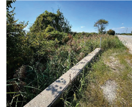
Photo 30: Culvert outlet at Crossing 6, south side of County Road 46.
