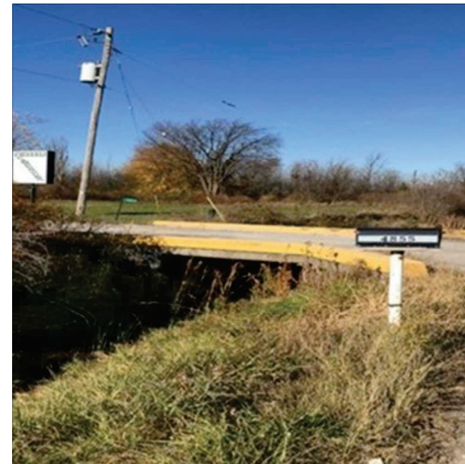
Photo 7: Watercourse Crossing 2 is conveyed under a concrete bridge culvert located north of the Highway 401 underpass.
