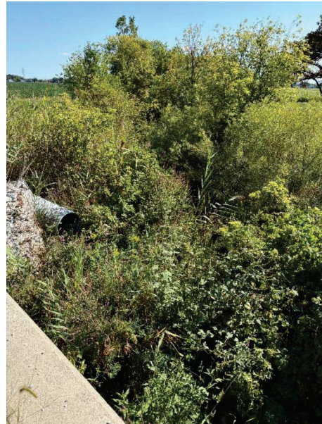
Photo 40: Facing south at Crossing 8, from south side of County Road 46.
