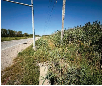
Photo 24: Facing west at Crossing 5, north side of County Road 46. Dry Channel.
