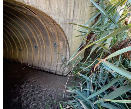
Photo 31: Facing southwest, at outlet of twin-barrel concrete pipe culvert at Crossing 6.
