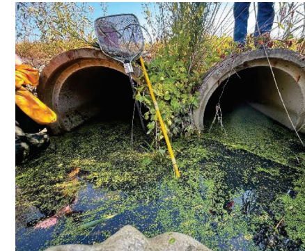
Photo 2: Facing north of twin concrete culverts at Crossing 1.
