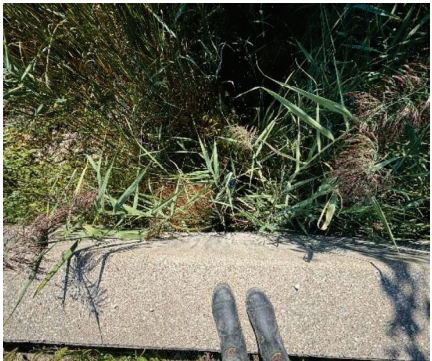
Photo 33: Birds eye view of channel south side of County Road 46.
