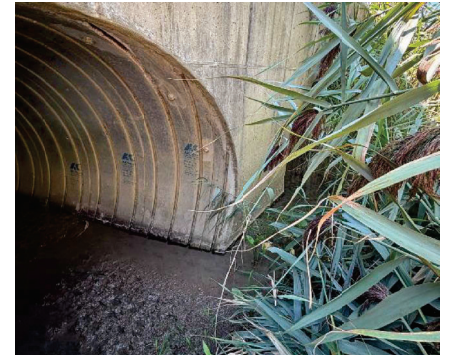
Photo 31: Facing southwest, at outlet of twin-barrel concrete pipe culvert at Crossing 6.
