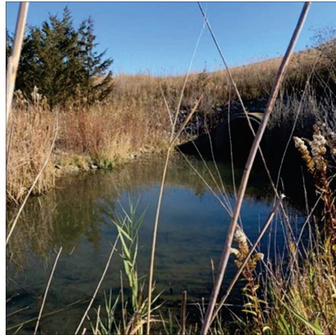
Photo 2: Culvert under Highway 401 overpass further west of Study Area, connected to Watercourse Crossing 1.
