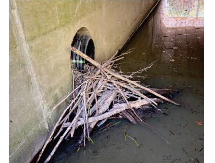
Photo 39: Habitat structure and Muskrat observed within concrete culvert at Crossing 7.
