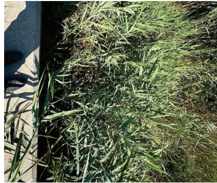
Photo 28: Culvert inlet at Crossing 5, south side of County Road 46.
