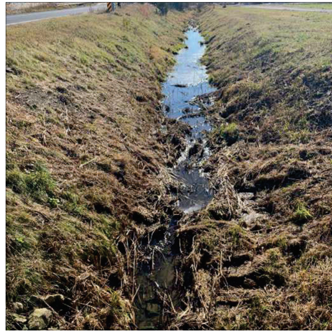
Photo 10: Watercourse Crossing 4, inundated ditch parallel to Concession Road 9.
