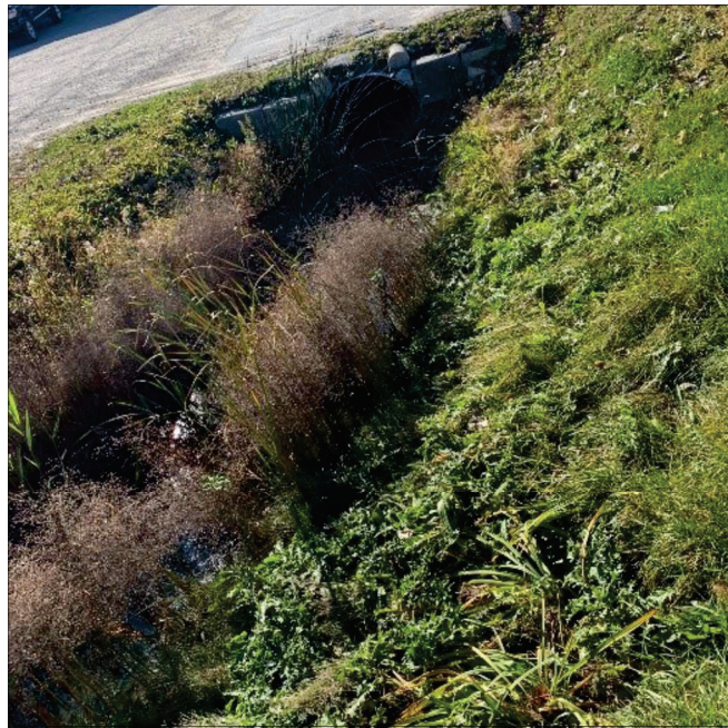
Photo 9: Outlet of forested ravine (Watercourse Crossing 3) inundates the linear ditch south of and parallel to CR 46.
