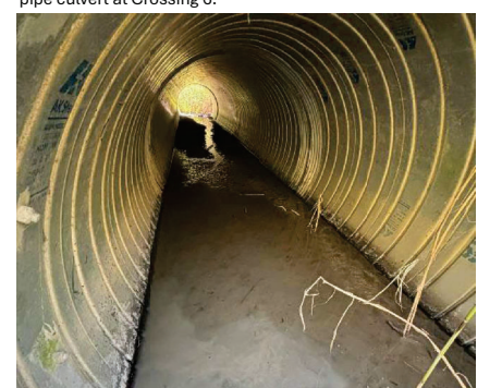
Photo 34: West barrel of concrete pipe culvert at Crossing 6 (facing south).
