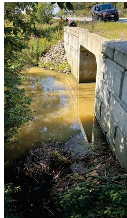
Photo 35: Inlet of concrete box culvert, facing west from south side of County Road 46.
