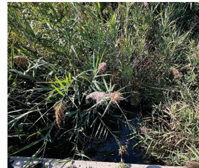
Photo 20: Culvert inlet at Crossing 4, south side of County Road 46.
