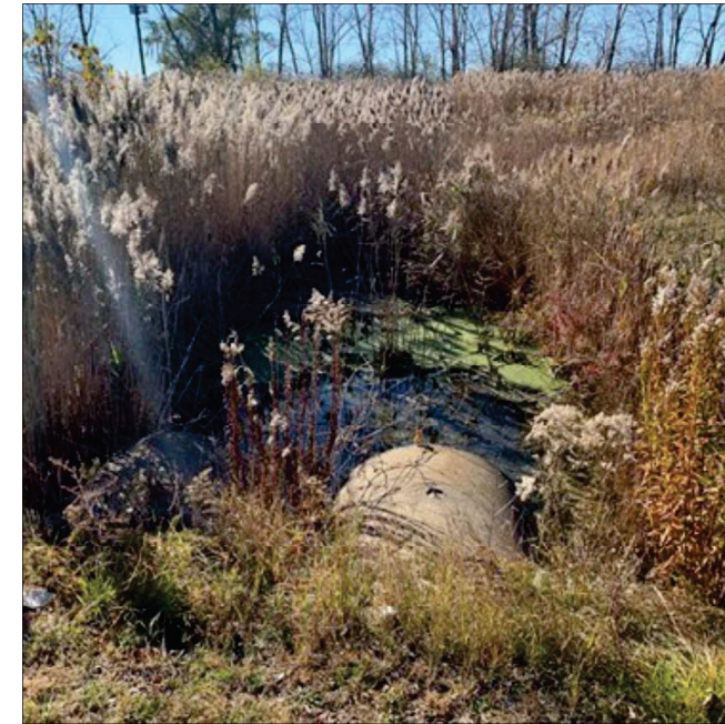
Photo 5: Culvert outlet of Watercourse Crossing 1, located south of CR 46.
