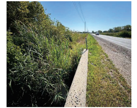
Photo 19: Facing east at Crossing 4, from the north side of County Road 46.
