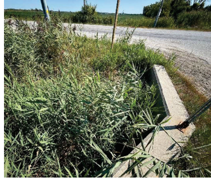
Photo 23: Facing northeast at Crossing 5, north side of County Road 46. Dry channel.
