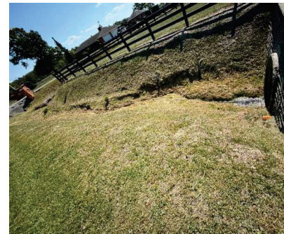
Photo 38: Ditch on south side of County Road 46, east of Crossing 7, confluent with the channel through the culvert pictured on far right.
