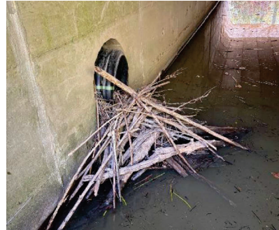
Photo 39: Habitat structure and Muskrat observed within concrete culvert at Crossing 7.
