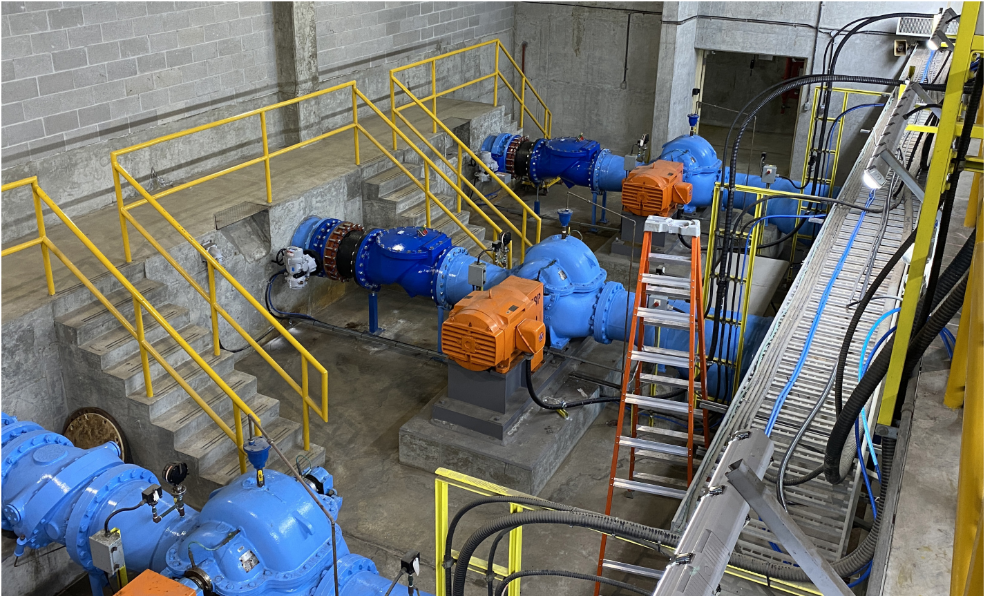
Backwash System Valve Replacements
