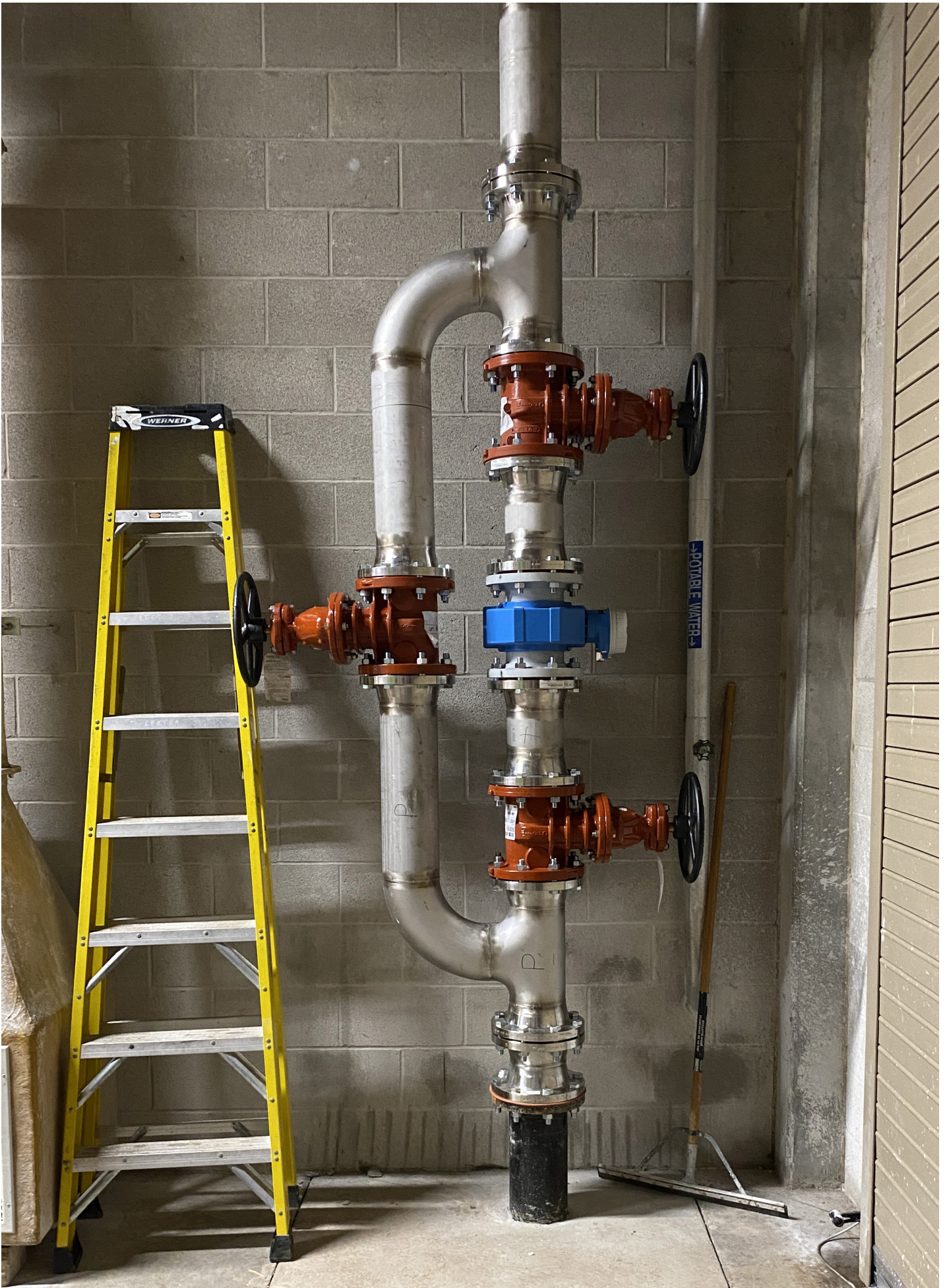
New Potable Water Feed to A.H. Weeks WTP
