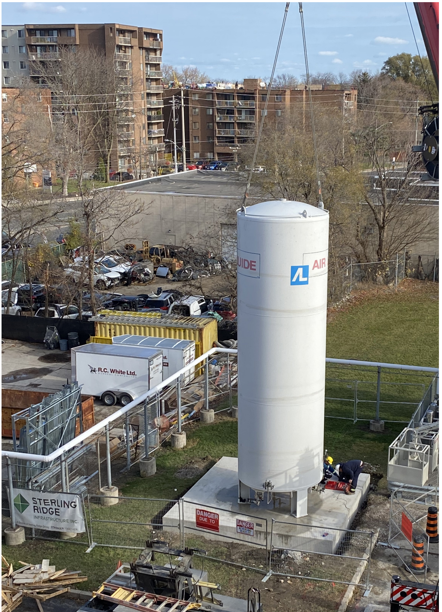
OWTP Decommission New CO 2 Tank Installation
