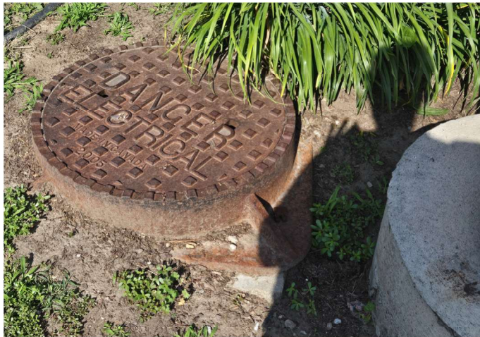
Figure 27: Traffic Manhole
