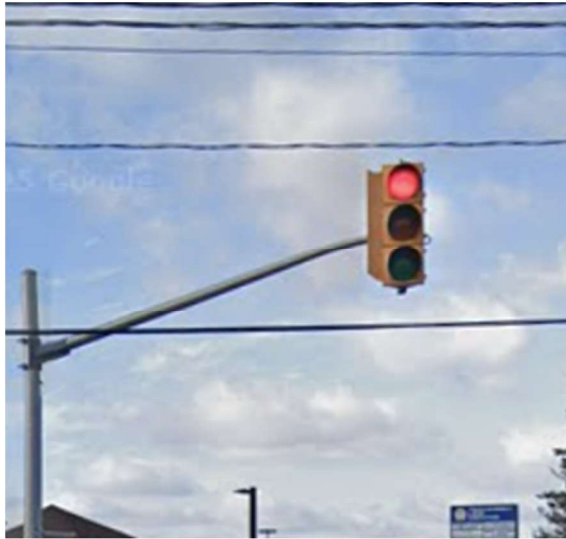
Figure 42: Traffic Signal Head Backboard
