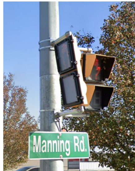
Figure 22: Pedestrian Signal Head
