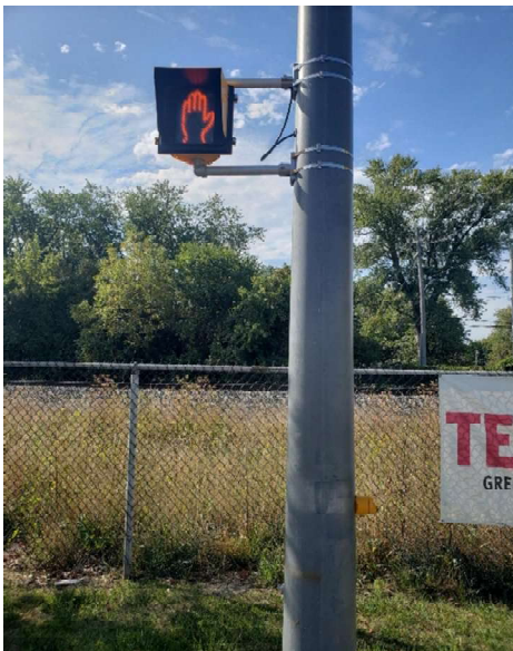
Figure 35: New Pedestrian Signal Head and Pushbutton
