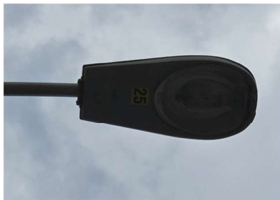
Figure 7: HPS Luminaire
