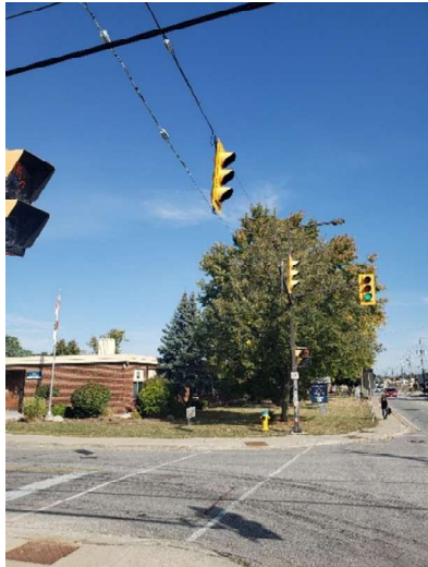
Figure 14: Overhead Span Wire
