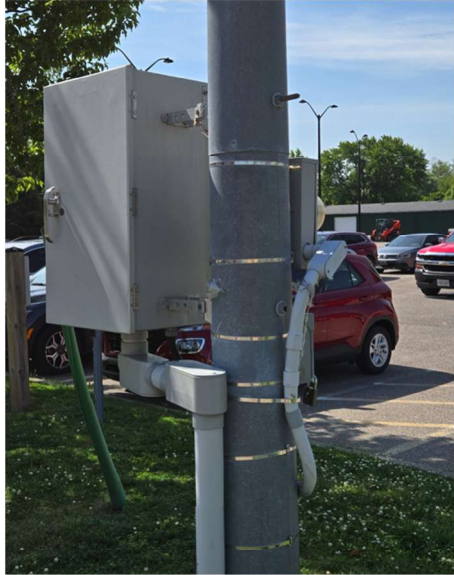
Figure 15: Damaged Conduit
