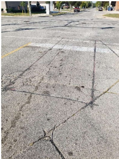
Figure 12: New Loops Installed
