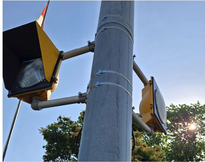
Figure 34: Pedestrian Signal Heads
