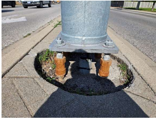
Figure 32: Traffic Pole Base and Anchor Bolts
