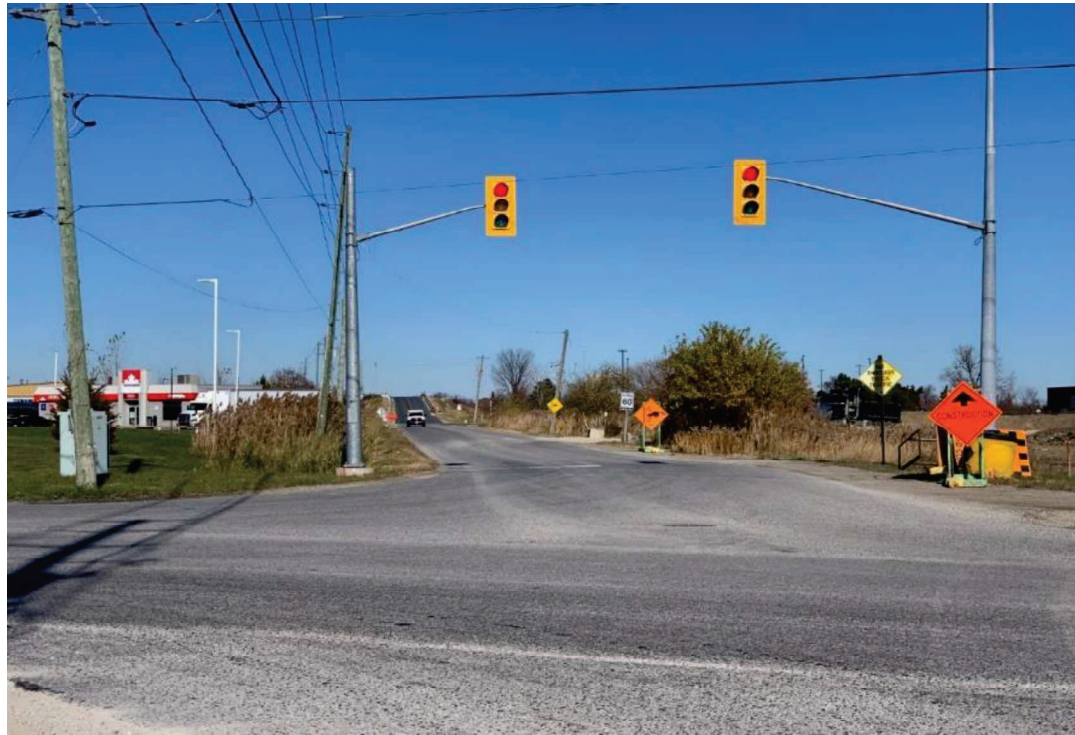
Photo 3: 8th Concession Road and County Road 46 intersection, facing north
