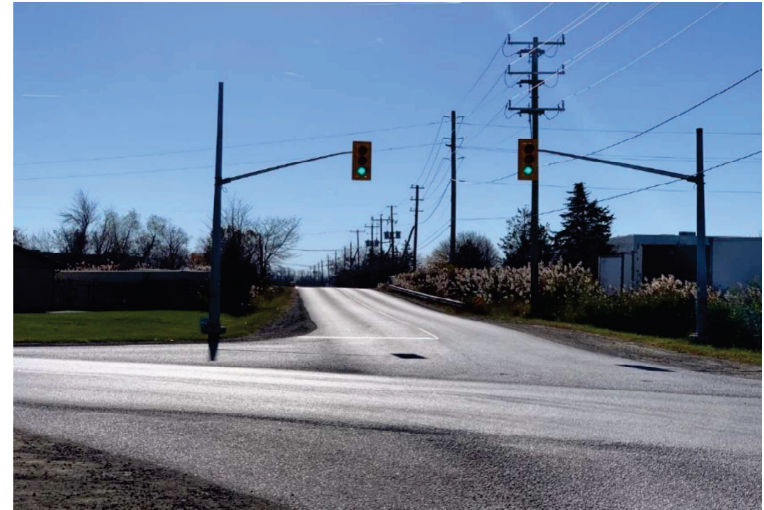
Photo 5: 8th Concession Road and County Road 46 intersection, facing south
