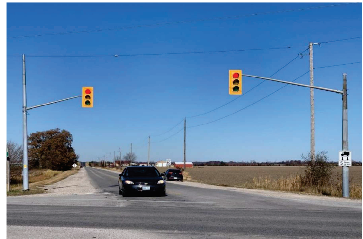
Photo 2: 9th Concession Road and County Road 46 intersection, facing north
