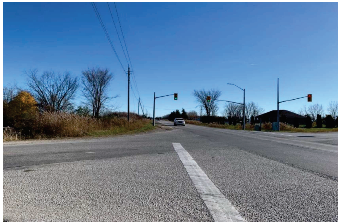
Photo 4: 9th Concession Road and County Road 46 intersection, facing east
