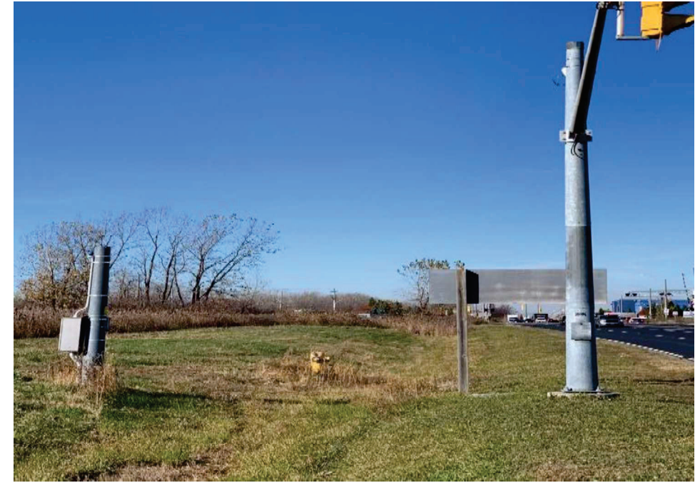
Photo 3: Highway 401 Westbound ramp terminal, facing west
