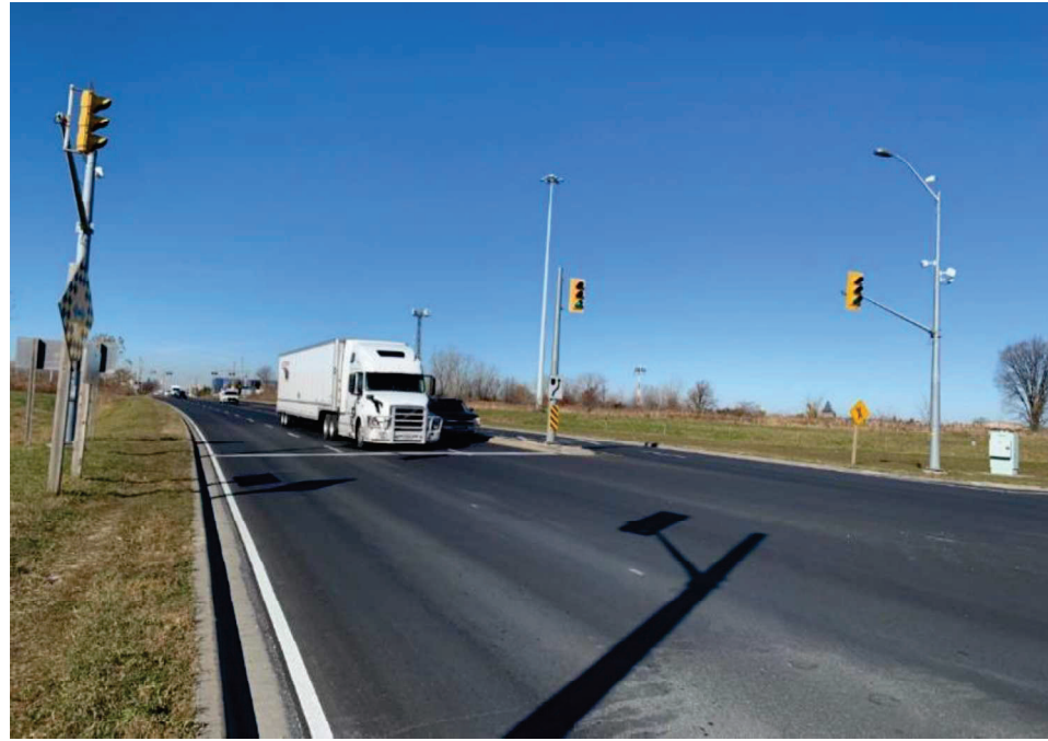
Photo 1: Highway 401 Westbound ramp terminal, facing northwest
