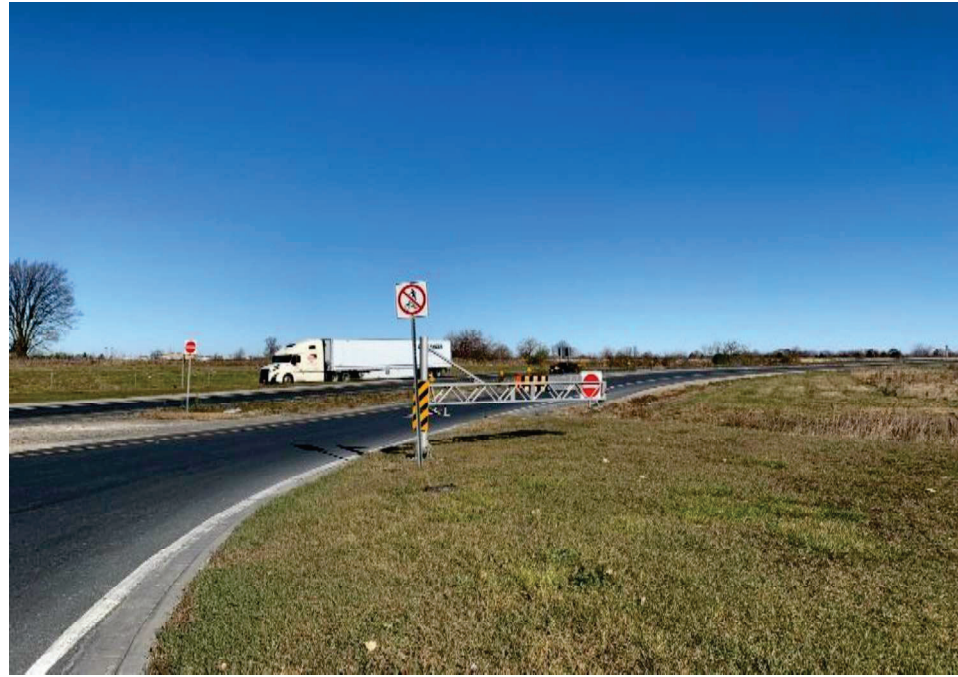
Photo 5: Highway 401 Eastbound on-ramp / eastbound ramp terminal, facing north
