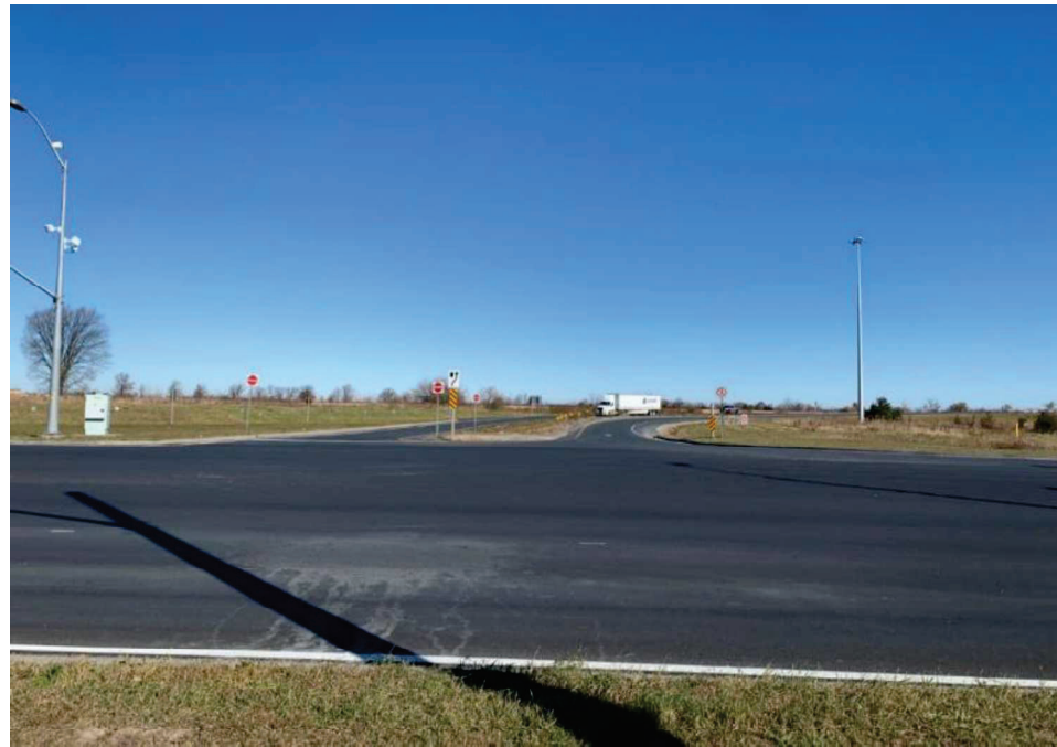
Photo 2: Highway 401 Westbound ramp terminal, facing north
