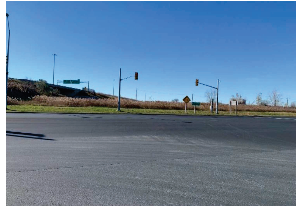
Photo 4: Highway 401 Westbound ramp terminal, facing south
